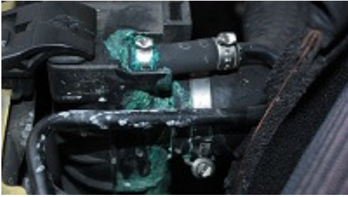
A severe coolant stain from a leak around a hose.
